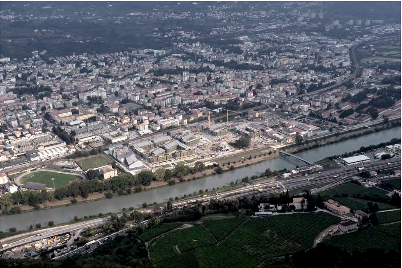
“Le Albero” in Trento, a new eco-neighborhood by Renzo Piano (Photographs by F. Cella)
