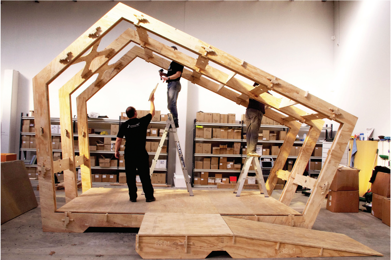
Fig. 1. Wiki House_Building the prototype. Source: http://spacecraft.co.nz/ .
