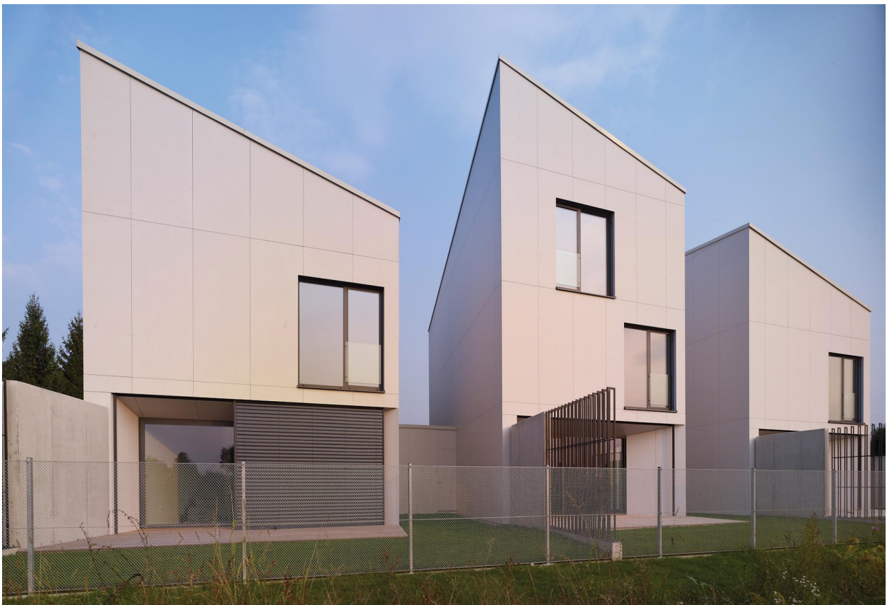
Cultural and Pastoral Centre of the Serbian Orthodox Church Parish in Ljubljana - Built: 2011 Architect: Atelje Neapolis: Borut Simič, Janez Žerjav - Location: Prešernova Street, Ljubljana
